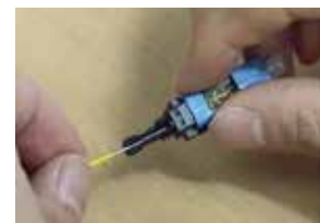
Insert the fiber into the connector body until the strand meets resistance and arches
